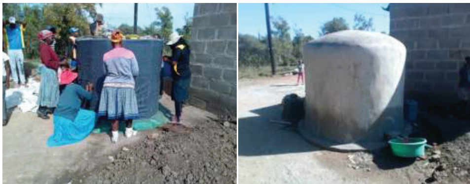
pictures: Concrete tank construction simplified by our staff under the Resilience project
